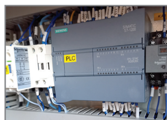
GESTIONE MACCHINA PLC SIEMENS MACHINE CONTROLLED BY PLC SIEMENS
